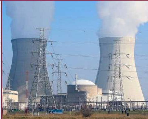
HIGH VOLTAGE 66kV to 132kV
